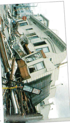
▲ Figure 5-32 Earthquakes can destroy homes and buckle roads.
