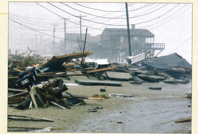
▲ Figure 8-28 Hurricane damage in Kitty Hawk, North Carolina
